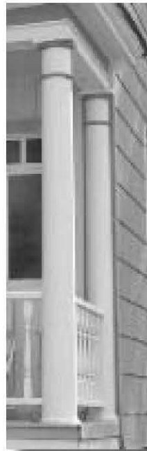
Simple, massive round columns and matching pilasters. Queen Anne free-classic style on Late Victorian dwelling.
