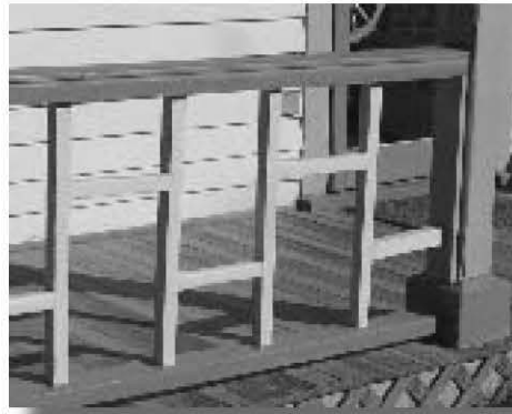
Simple, square vertical balusters and horizontal members, beveled rails and chamfered posts. On Folk Victorian dwelling.
