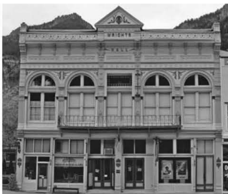
Wright Opera House - 1888 460 Main Street double storefront
