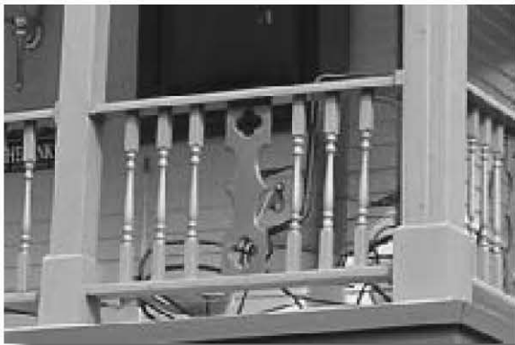
Chamfered square posts with square bases. Both turned spindlework balusters and scroll-sawed, flat centered baluster. On Late Victorian dwelling.
