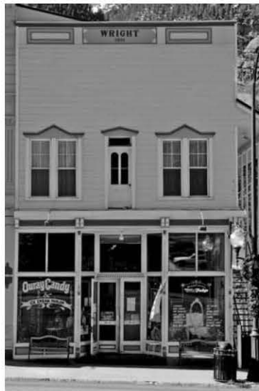
Wright Building 480 Main Street 1881
