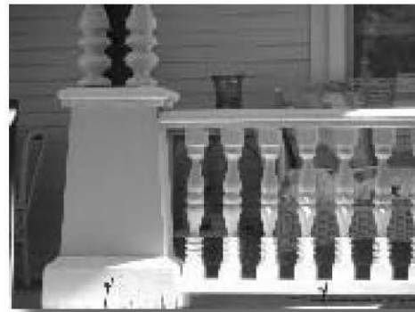
Elaborate spindlework balustrade and paired turned posts on tapered bases. On Late Victorian dwelling.
