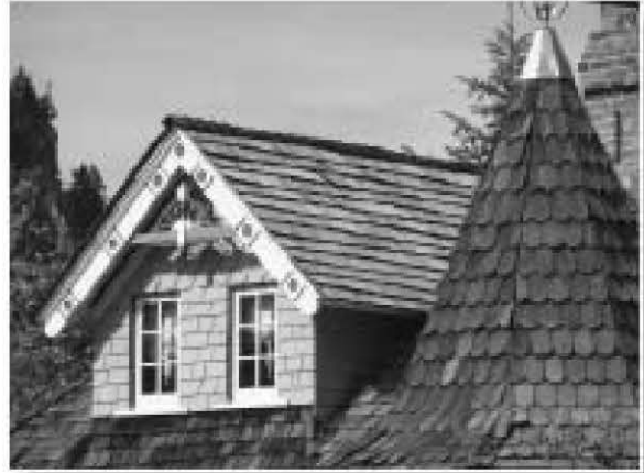
Gabled double-window dormer with ornated gable truss and bargeboard. Both square and beveled shingles and six-light windows.
