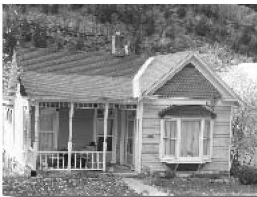
830 4th Street Partial front porch with two transomed entries in ell. Turned posts supporting a shed roof. Spindlework frieze and spindle balustrade. On one-story, front-gabled frame dwelling.
