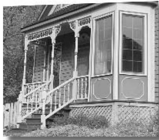
727 4th Street Shallow, partial front porch with turned posts supporting a half-hipped roof, sheltering a beveled bay with 10-lite windows.
