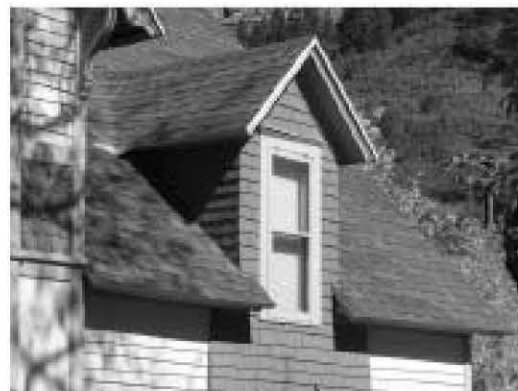
Gabled wall dormer. Note dormer sidewalls.
