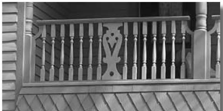
Turned spindlework posts and pilasters. Both turned spindlework balusters and scroll-sawed, flat centered baluster. On Queen Anne style dwelling.
