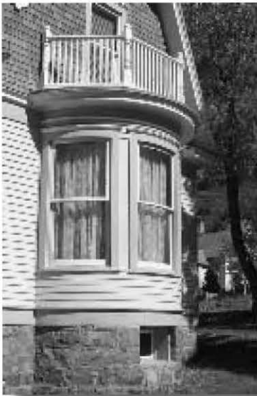
Flat-roofed semi-circular bay window with 1-over-1 units; topped by a simple balustrade
