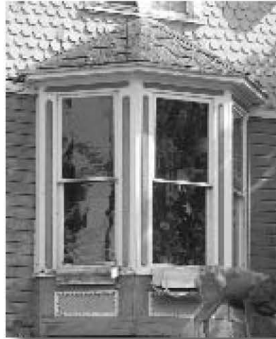
Beveled bay window with a hipped roof and 1-over-1 windows.
