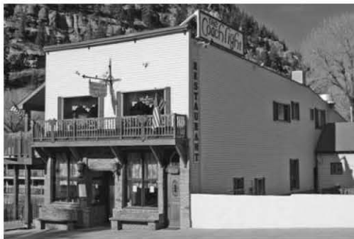
Belvedere Hotel c1900 118 7th Avenue Nineteenth-Century Commercial building
