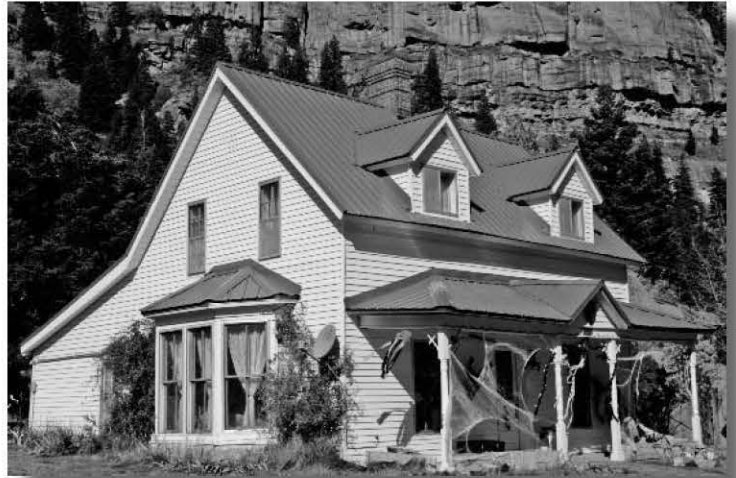
McIntyre - Wright House 442 Oak Street 1878
