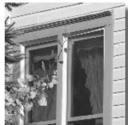
Paired 1-over-1 windows with simple beveled hood mold to shed rain.
