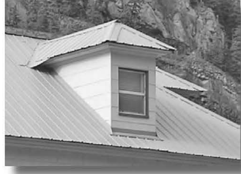
Half-hipped dormer on American Foursquare roof.
