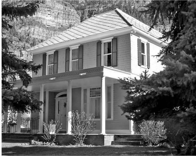
Haskins – Mostyn – Franz House 431 4th Street 1908 est.
