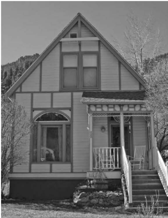
Biddlecom House 322 Oak Street 1889
