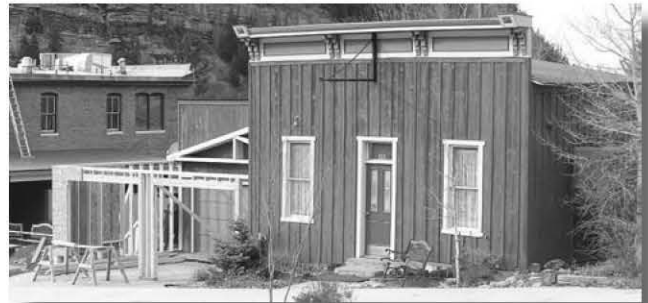
Reed Assay Office, Rathmell Abstract Office 1883 332 5th Avenue False-Front Commercial building
