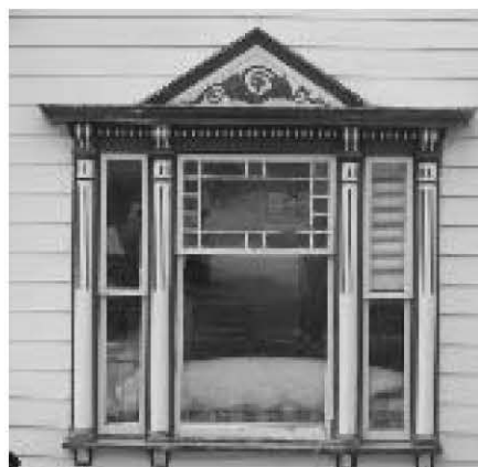
Pediment with brackets above tripartite window with glazed multicolored lites above center window and narrow double-hung windows.
