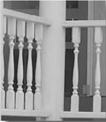
Square post with turned spindlework balusters.
