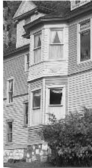
Two-story, beveled bay with 1-over-1 units above and below. Lower windows pedimented. Upper unit shingled with diamond ornamentation. Hipped roof.
