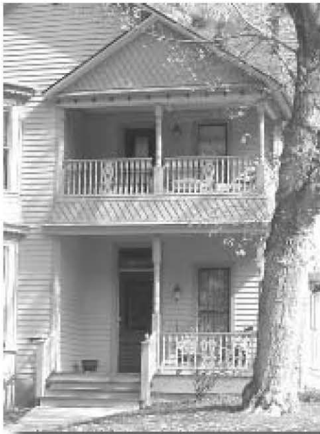
429 5th Street An inset partial double porch is beneath front gable. Turned posts and spindlework balustrades. On two-story frame cross-gabled dwelling.
