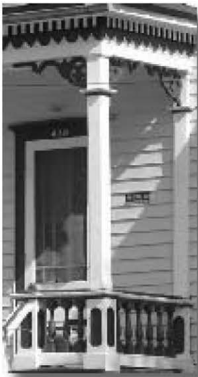
Square columns and an elaborate frieze of scalloped and dentil ornamentation. Pilasters on wall. Italianate style building
