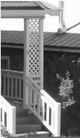
Doubled square corner posts with lattice between. On Late Victorian dwelling.
