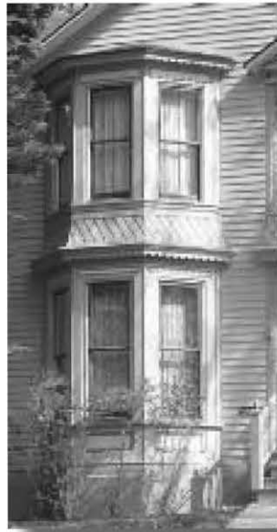
Two-story flat-roofed, beveled bay window with 1-over-1 windows and diamond-shaped shingle trim.
