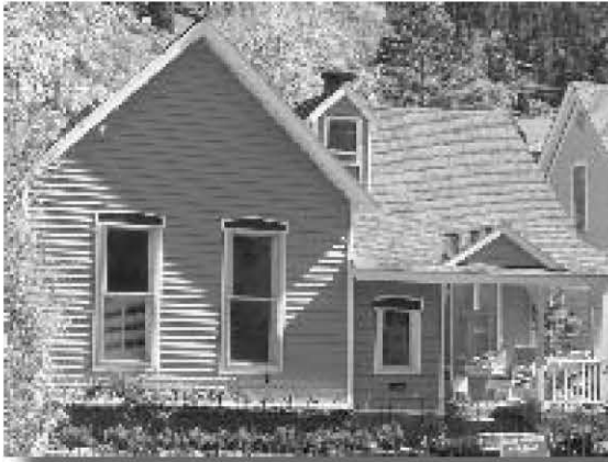
629 4th Street Partial porch in ell with columns supporting a shed roof, a plain balustrade, brackets, and pediment over entrance on a 1-1/2-story, cross-gabled frame dwelling.
