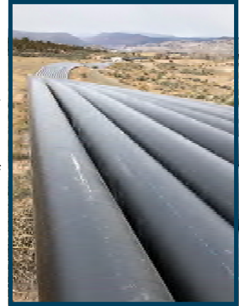
15,000 L.F. 18" Diameter Fusible PVC Gypsum, CO
