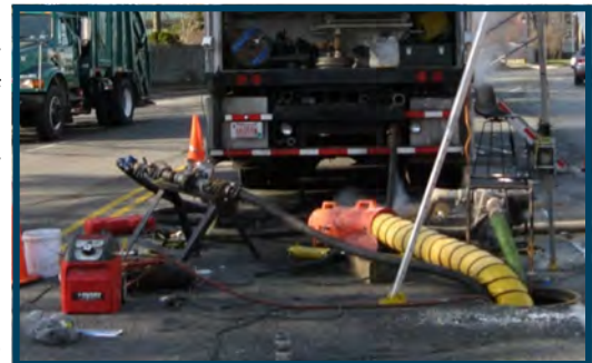
Cure in Place Pipe Installation—Denver Metropolitan Area
