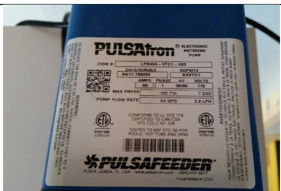
Figure 4. Chemical Metering Pump
