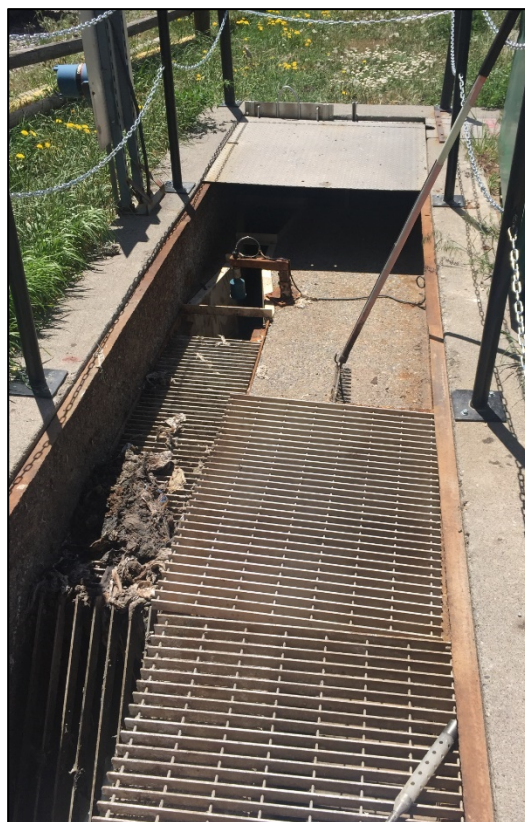
Figure 7. Existing Screening
