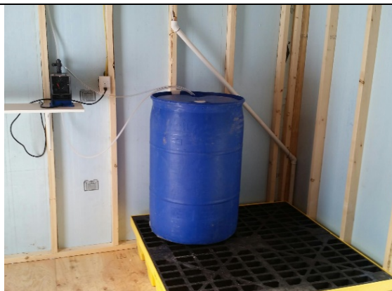
Figure 2. Sodium Hypochlorite Feed Tank
