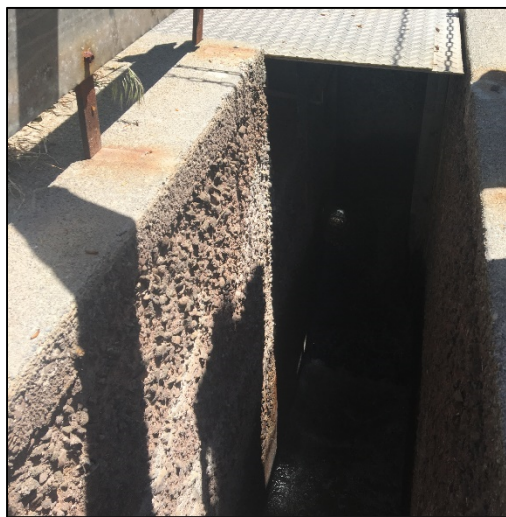
Figure 8. Existing Influent Grit Chamber
