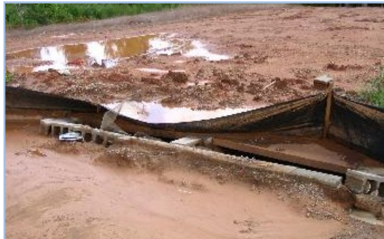
FAILING SILT FENCE
