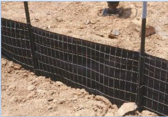
PROPERLY INSTALLED SILT FENCE
