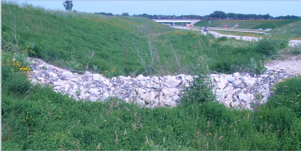
PERMANENT STONE DITCH CHECK
