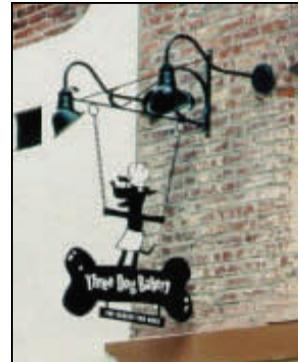
clearance of 12 inches between the building face and sign and maintaining a projection of 36 inches.
