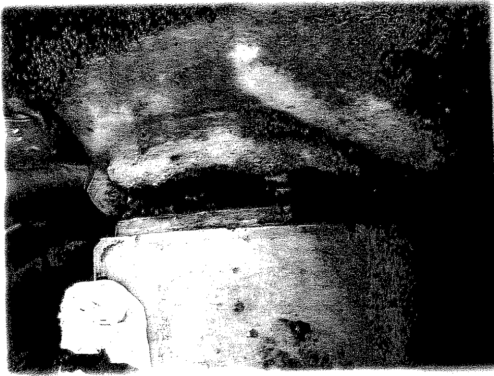
Leak in primary effluent line was detected on west side of Primary Clarifier #2 where drop box pipe ties into the tee and August Winter cleaned out joint.
