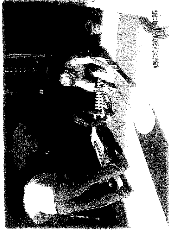
Faith working on wiring automated valves for the aeration tanks and Miron laying concrete around wiring for the future MCCs.
