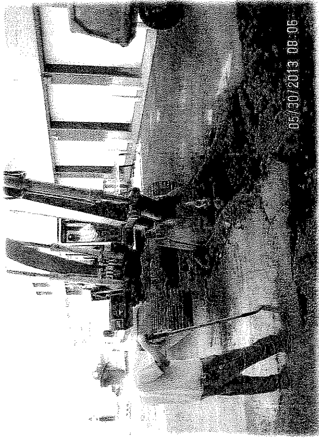
Miron prepared the sidewalk underneath the south blower building's heat exchangers and August Winter worked on excavating for 8" PVC centrate drain line.
