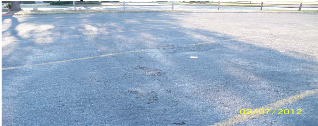
Sample pothole area that will require saw cutting and subgrade stabilized prior to recoating.
