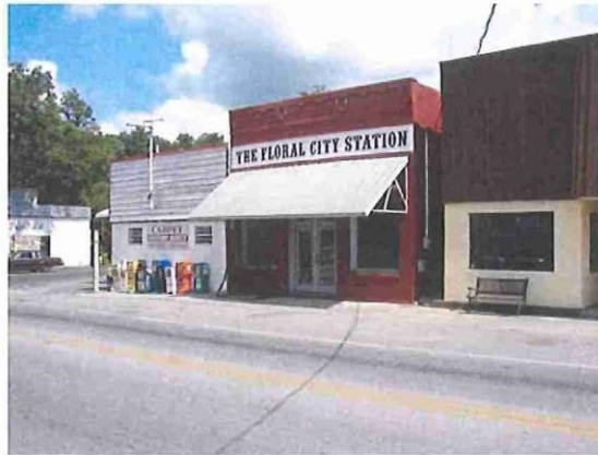
“Old Bank Building” in Floral City – Early 20 th Century Storefront Style
