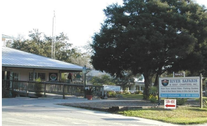
Nonresidential Stemwall Construction
