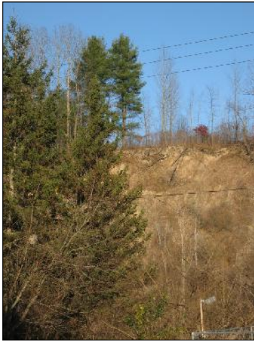
Figure 7: Steep Slope, Route 13
