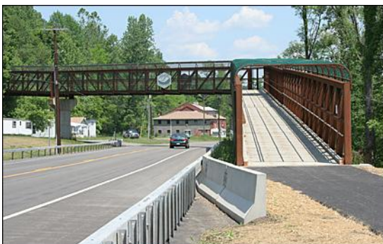
Bridge over State Route 14 in the Town of Veteran along the Catharine Valley Trail.
