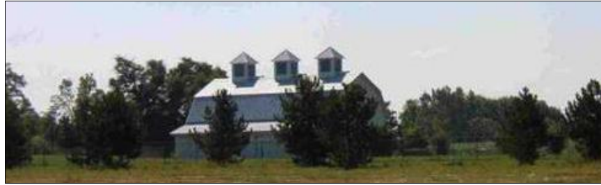
Source: Patrick O'Dell, National Park Service, disguised compressor site
