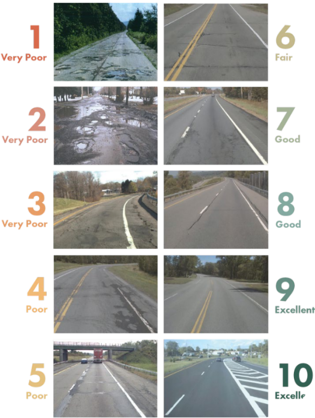
Figure 5.5 Examples of Pavement Condition
