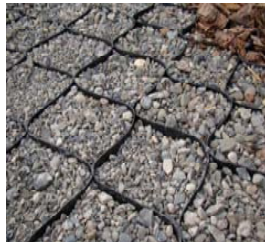
Geoweb—around the rain garden. Red chips accent the path
