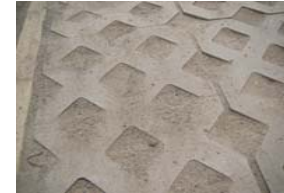
TURFSTONE was used for the picnic table pathway
