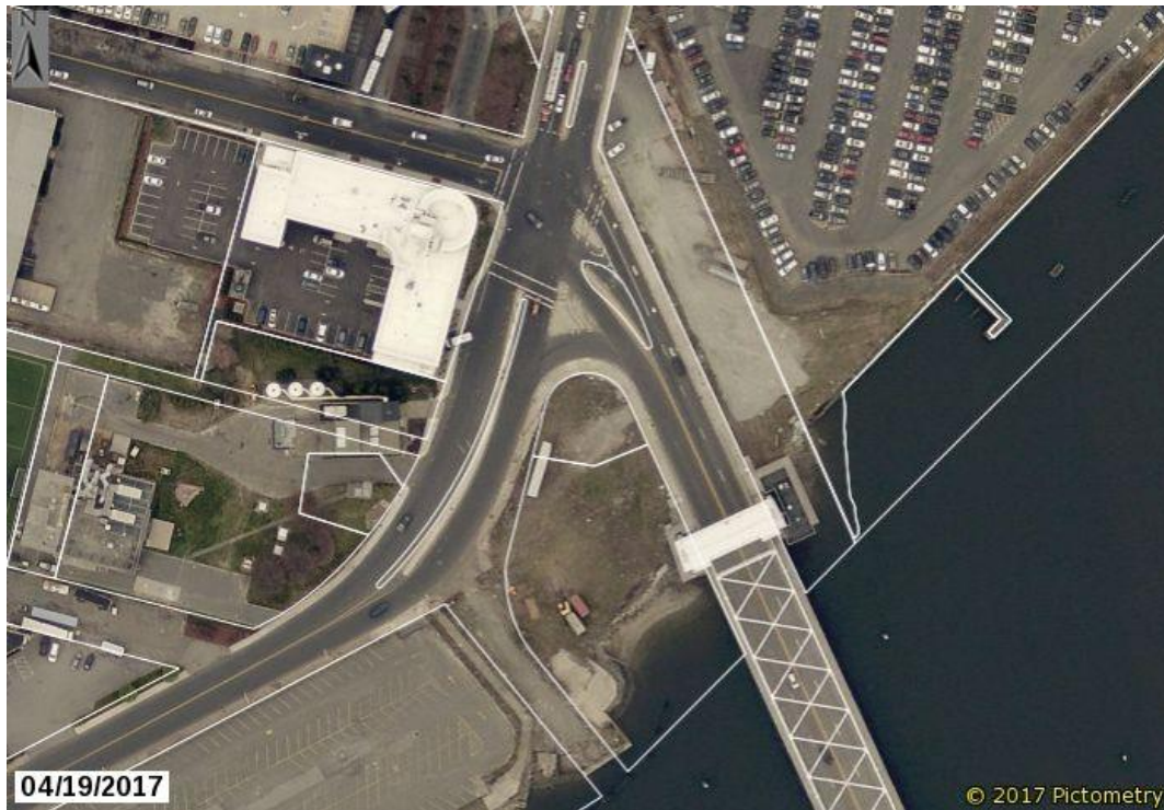
Figure 33: Aerial View of Parcels Adjacent to the Chelsea Street Bridge
