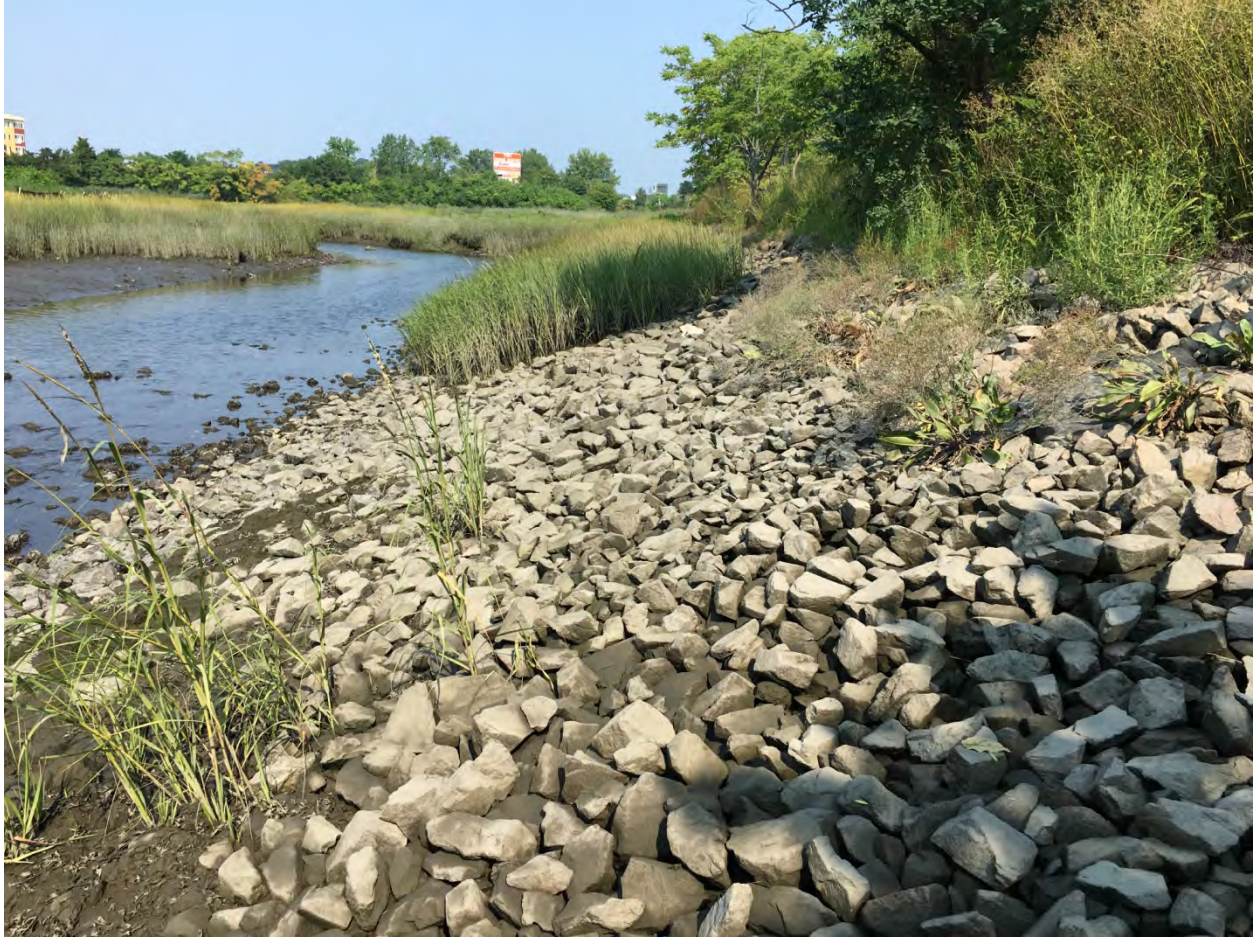
Photo 19. Riprap Upstream of Broadway Bridge on Northeast Bank
