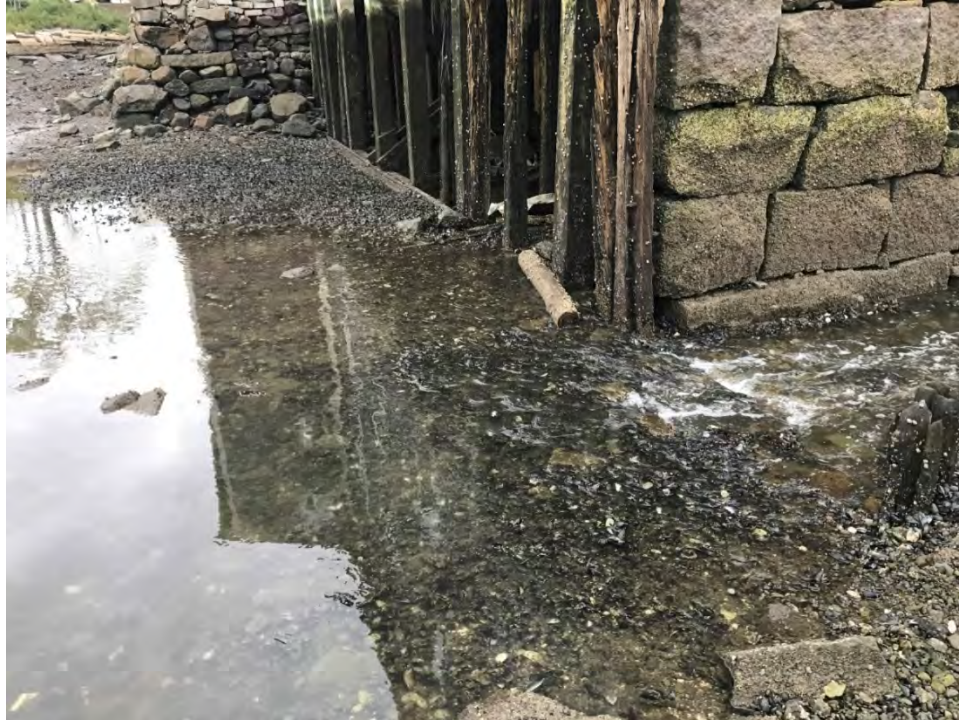
Photo 4. Low Level Flow Obstructions Beneath Mill Building
