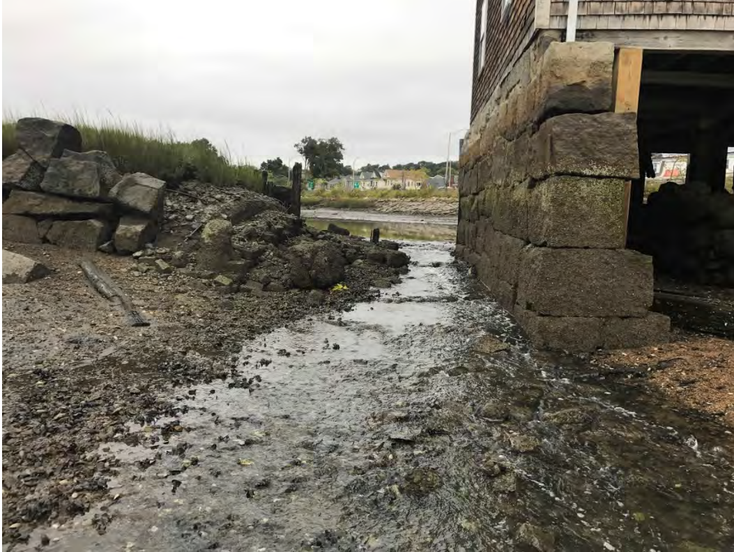
Photo 6. Primary Cut in Spice Mill Earthen Dam
