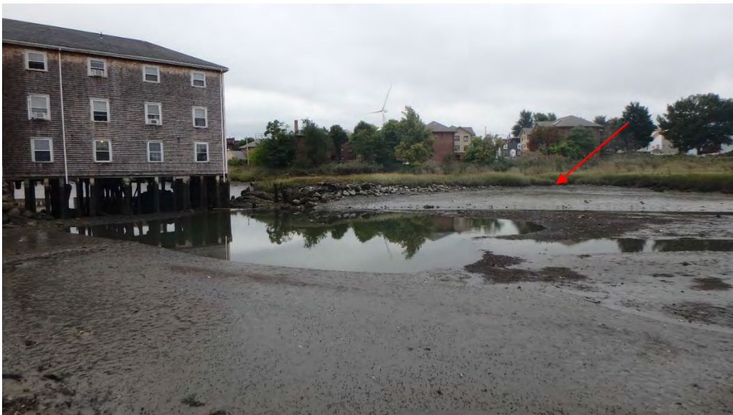
Photo 7. Secondary Cut in Earthen Dam (red arrow)
