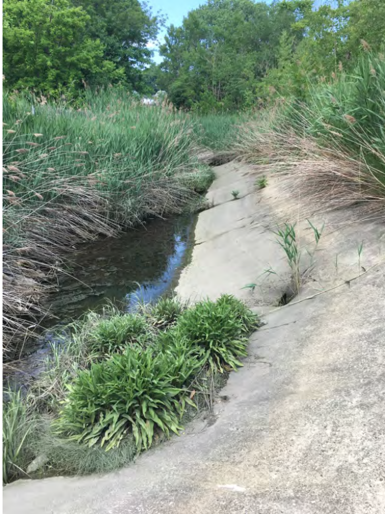
Photo 25. Concrete Revetment on South Bank of Tributary Channel
