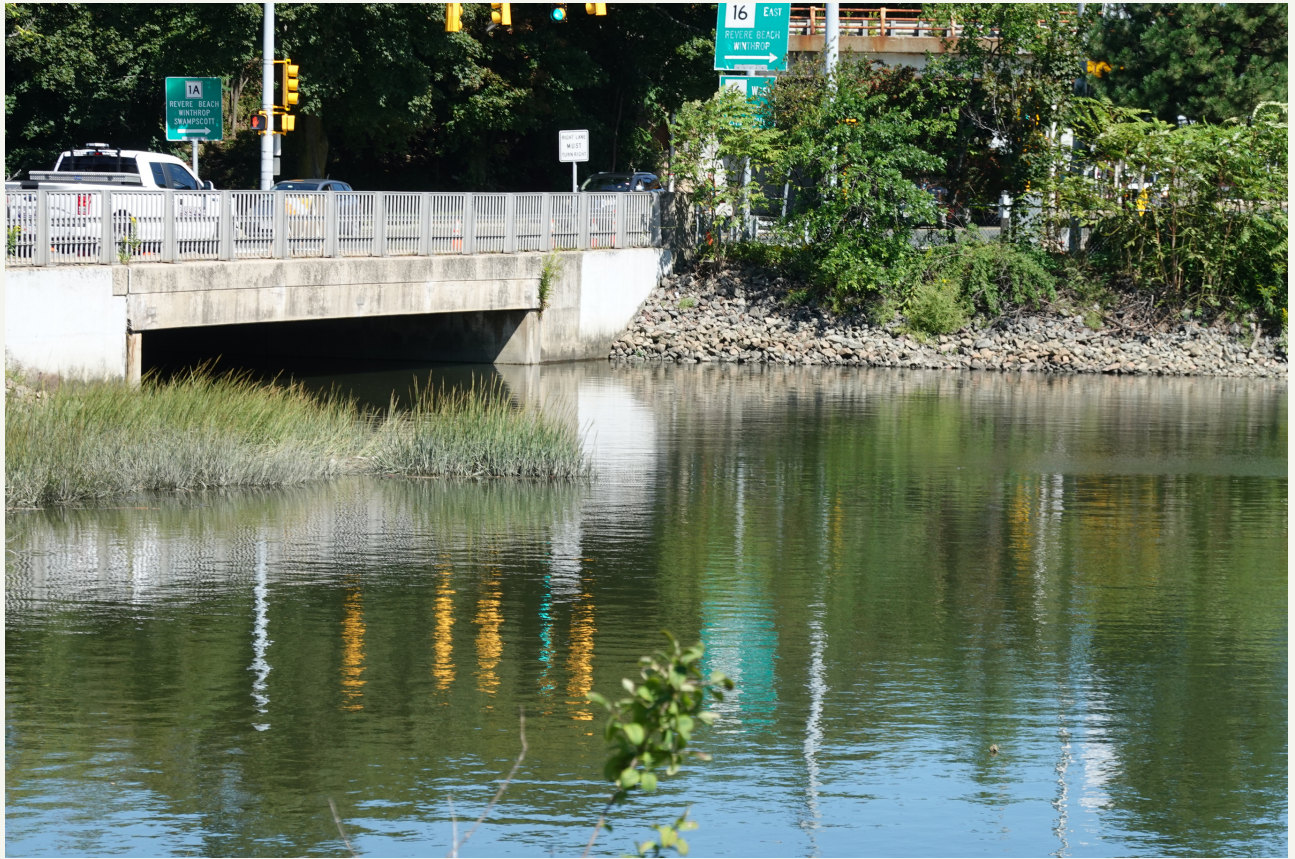
Chelsea Mill Creek: Broadway Bridge
