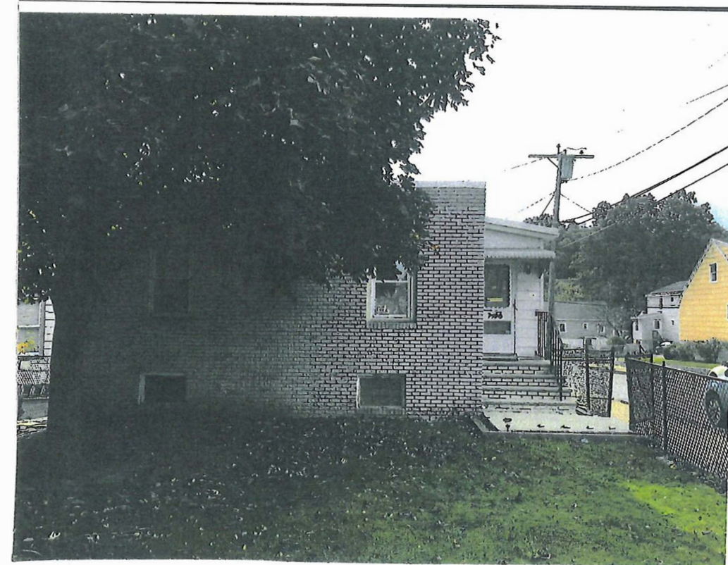
EXISTING LEFT SIDE – 30 PROSPECT AVE.
