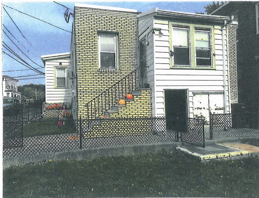
EXISTING RIGHT SIDE – 30 PROSPECT AVE.
