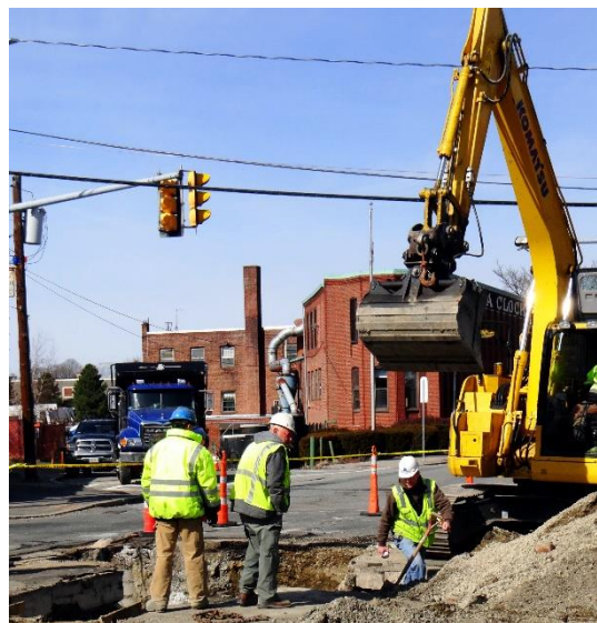
Workers replace water & sewer lines at the intersection of Everett Avenue & Carter Street.
