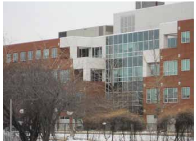
Approximately 1,200 employees work in the MITC building just beyond 5th & Chestnut.
