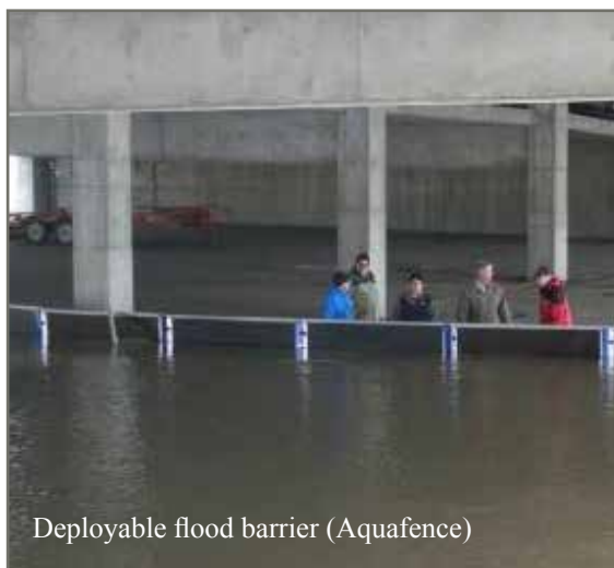
Example of a deployable flood wall. Metal panels could be a good option for future adaptation (EKO Flood USA).
