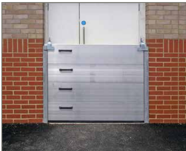
Example of a permanent perimeter wall (Stantec, Santa Barbara, CA - top) and flood logs (Flood Control International - bottom)
