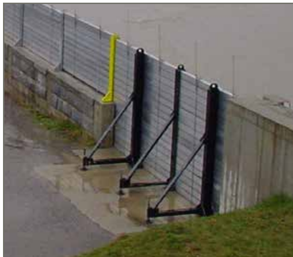
Example of a combination permanent and deployable wall along the waterfront (image from EKO Flood USA)
