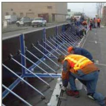
Aquafence Installation in Mount Vernon, WA
