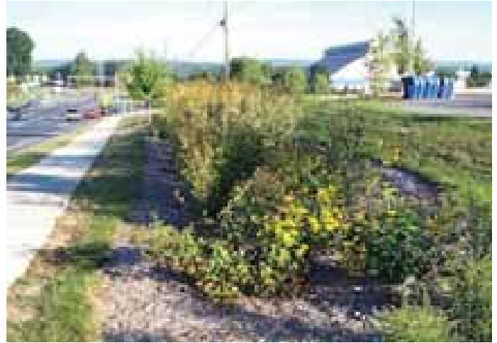
bio-retention swale example
