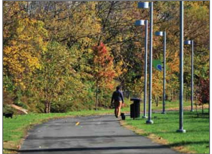
Asphalt Surface Trail
