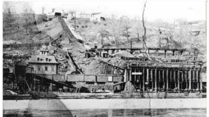
View of canal boat loading docks from Lehigh River
