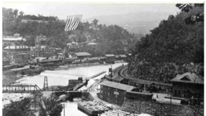
View of canal lock 1
