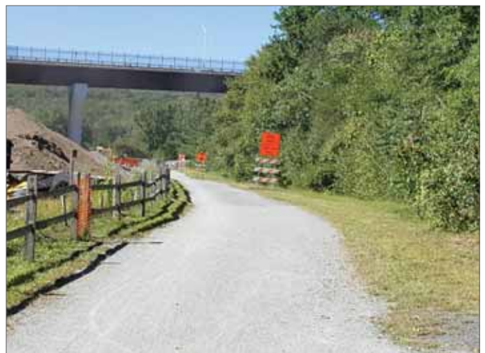
Compacted Aggregate Surface Trail
