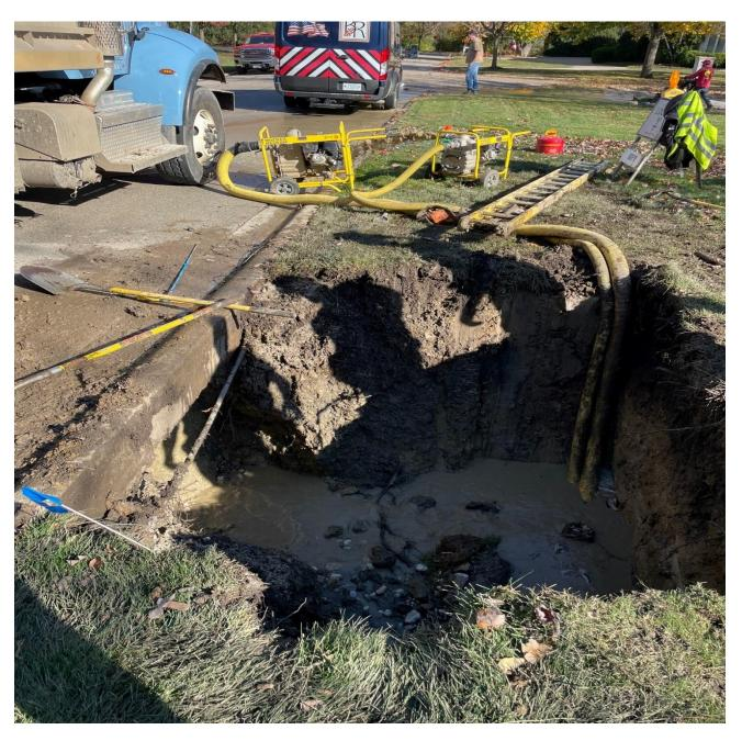
Replacing water main for reliability and fire safety.
