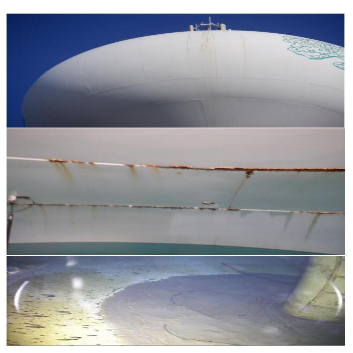
Recoating corroded surfaces of our South Water Tower.
