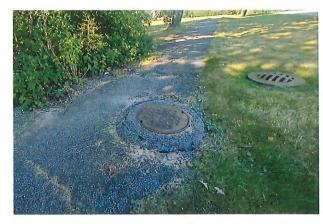
Figure 1 - View of significant trip hazard caused by the existing path settled around a sanitary structure.
