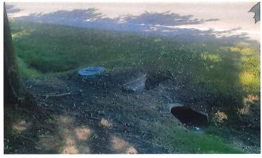
Figure 3 – Existing ditch and structure on-site exhibit erosion of sideslopes and exposed concrete.
