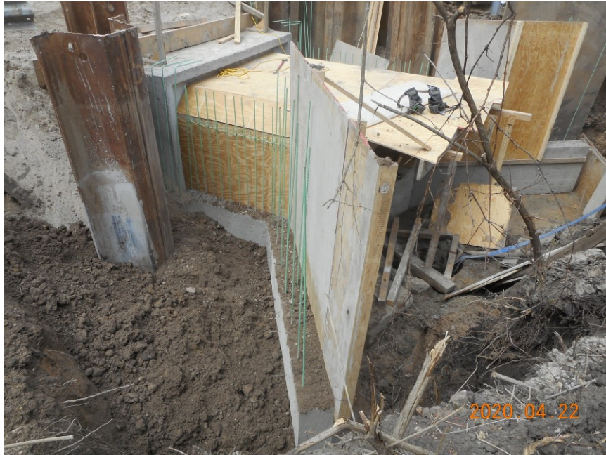
Exhibit 1 - Rebar erection and concrete forms to cast headwall, wingwalls, and connection to precast box section
