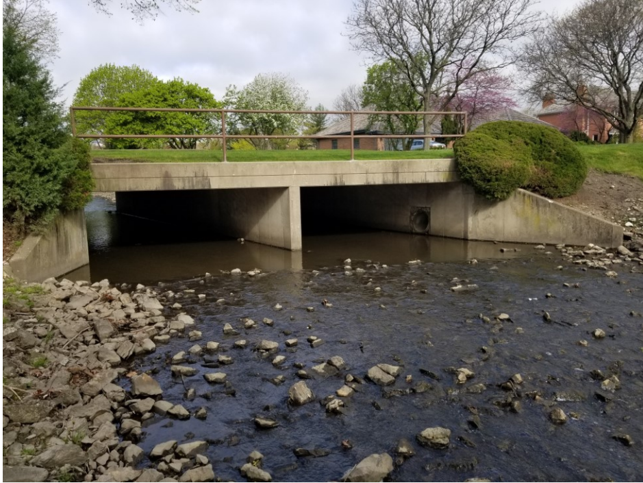
Exhibit 5 – 63 rd Street Ditch at Tomlin Drive, 2 – 5' x 13' Box Culvert
