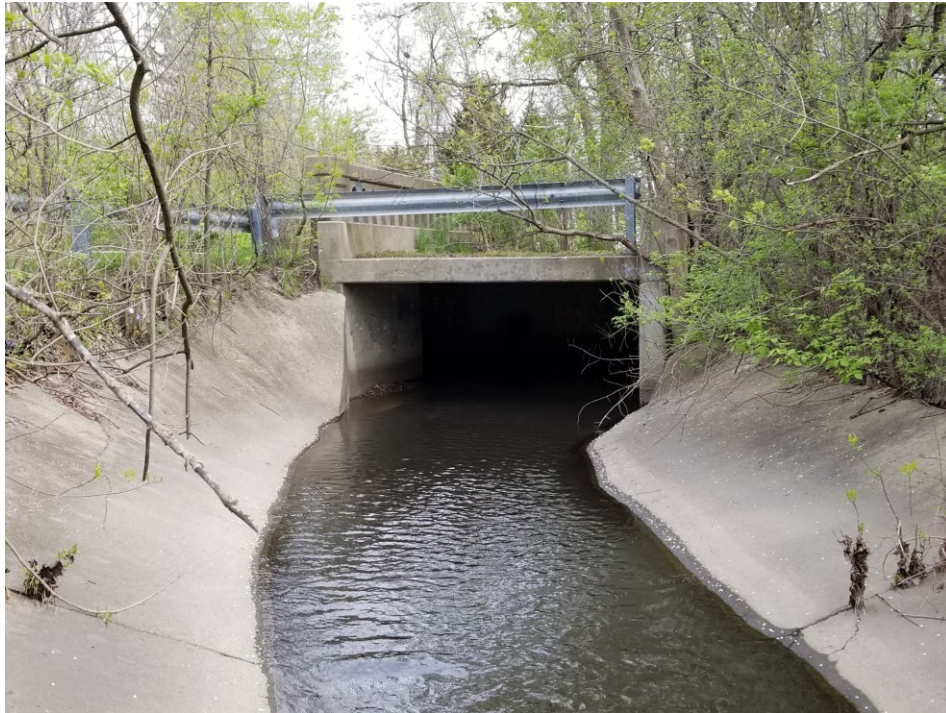
Exhibit 3 - 63 rd Street Ditch at Garfield Avenue, 5' x 12' Box Culvert
