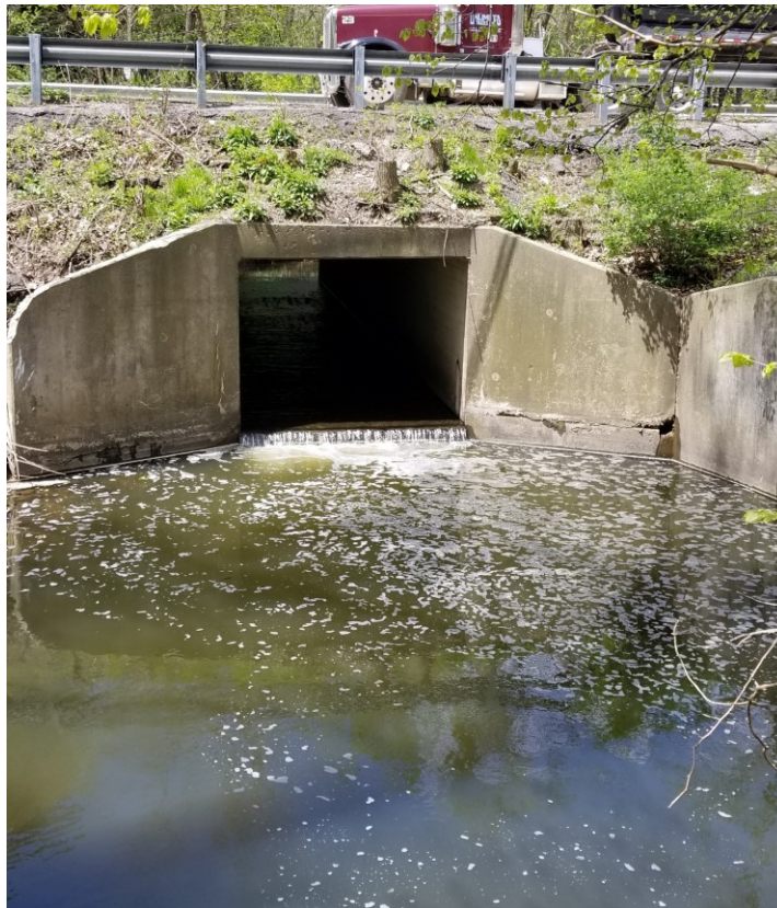
Exhibit 4 - 63 rd Street Ditch at County Line Road, 6' x 8' Box Culvert
