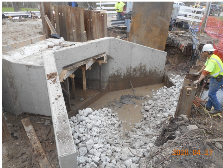
Exhibit 2 - Cast headwall, wingwalls, and connection to precast box section
