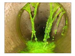
sanitary sewers to quantify the amount of dyed water infiltrating into the sanitary sewers.
