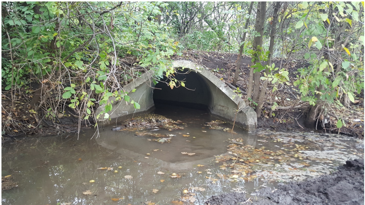
AFTER: Culvert Discharge – Grate Removed
