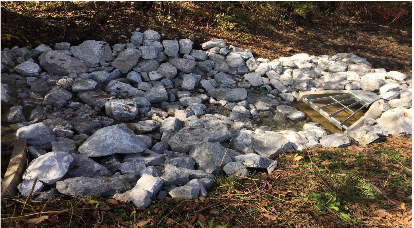
Pipe Outfall (18" RCCP w/6" PVC to Old CMP)
