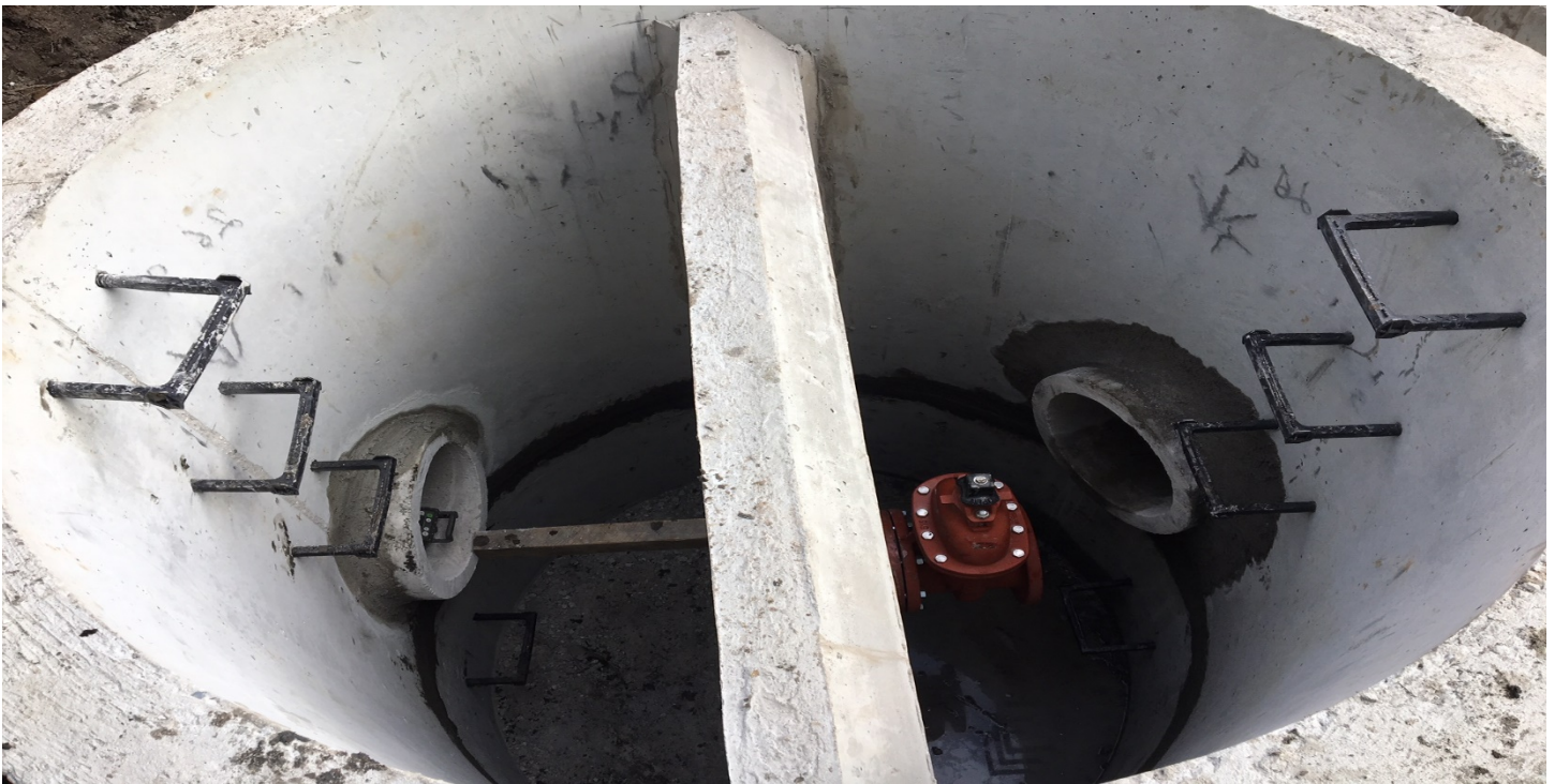
Control Structure, Internal Piping (Outfall to the Right)
