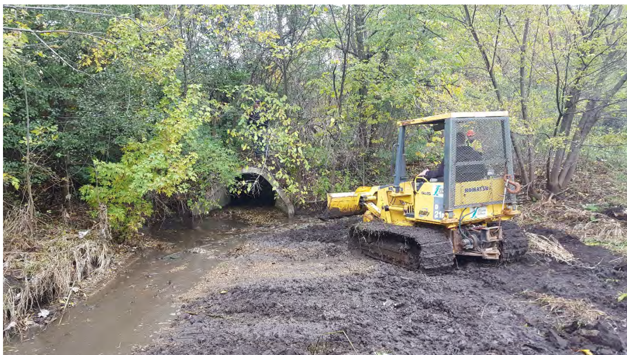
Culvert Pipe Discharge – Grate Removed & Ditch Re-Graded
