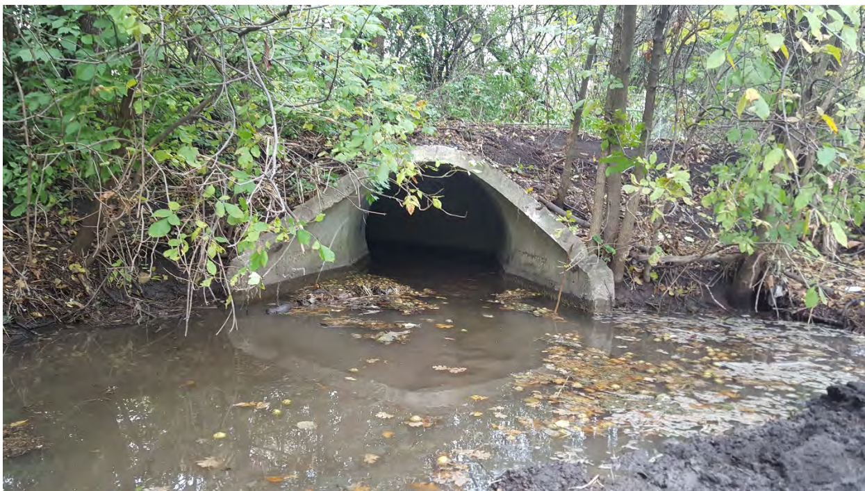
Culvert Pipe Discharge – Grate Removed
