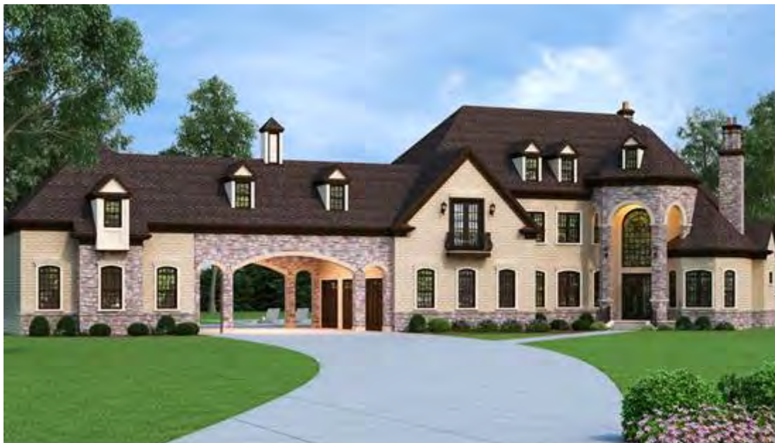
An example of a garage attached by a horizontal structural element or roof. An internal wall or party wall is not shared.
