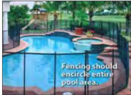
Like other pool fences, mesh fences should be a minimum of 48" in height. The distance between vertical support poles and the attached mesh, along with other manufactured factors, should be designed to hinder a child's ability to climb the fence. The removable vertical support posts should extend a minimum of 3 inches below grade and they should be spaced no greater than 40 inches apart. The bottom of the mesh barrier should not be more than 1 inch above the deck or installed surface.
