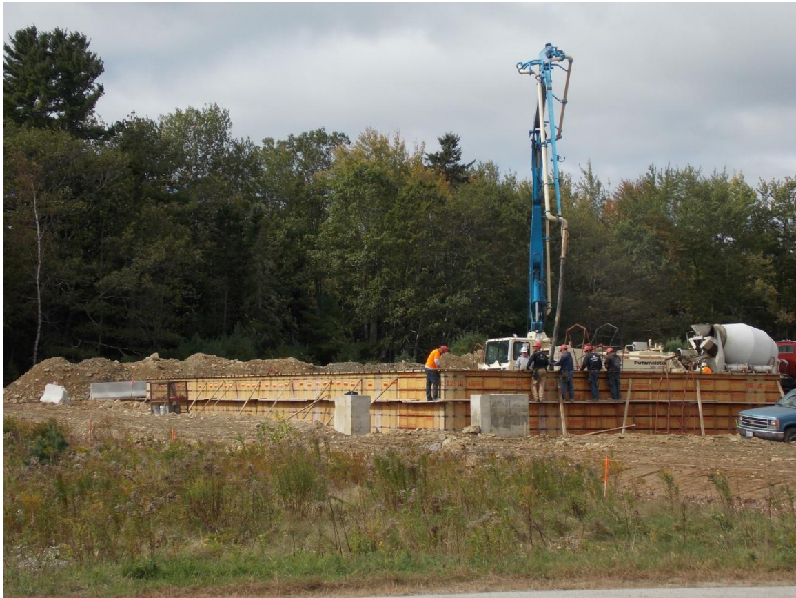
Pouring the foundation for the new Central Maine Cold Storage building within the Buckstown Heritage Park.
