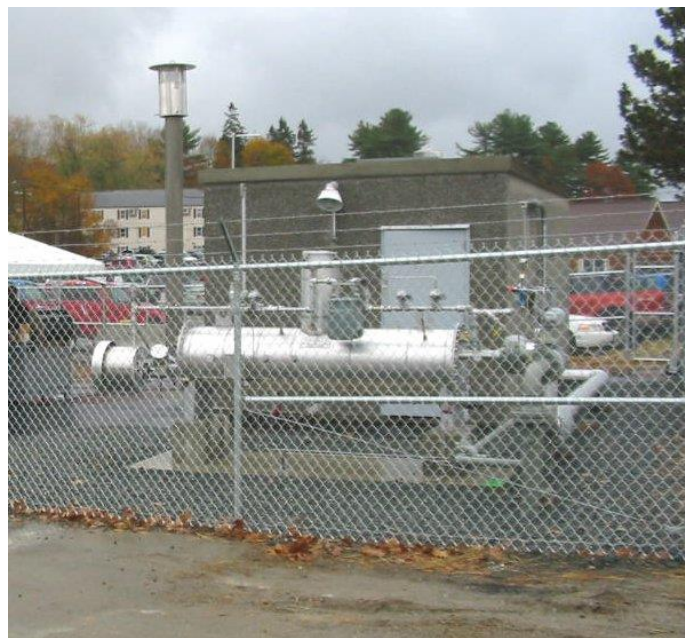
2013 Natural Gas Pressure Reduction Station at 3 River Road serving downtown Bucksport businesses & residences.
