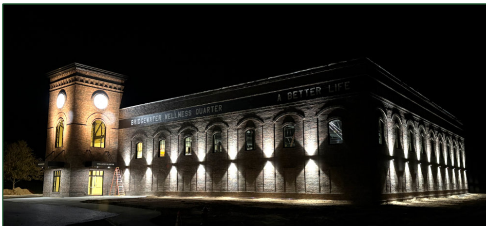
A view of the nearly completed Wellness Quarter at night.
