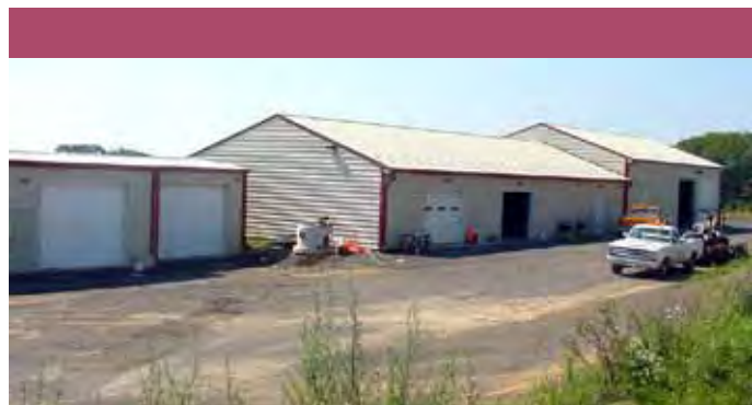
A new maintenance shop was constructed in 2003 on the east end of town. It is out of the flood plain and provides space for town equipment and supplies.
