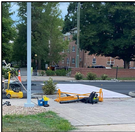
Asphalt stamping crosswalks on Dinkel Avenue in 2021.
