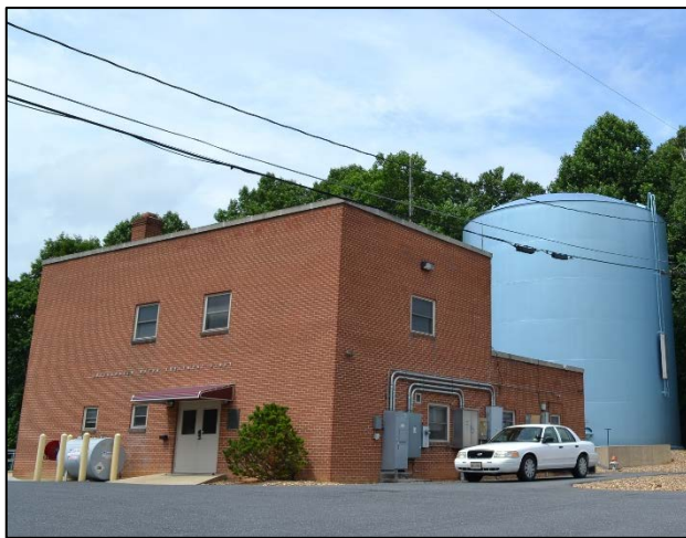
Bridgewater's Water Treatment Plant
