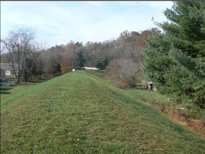
A portion of the levee on the northwestern portion of Town.
