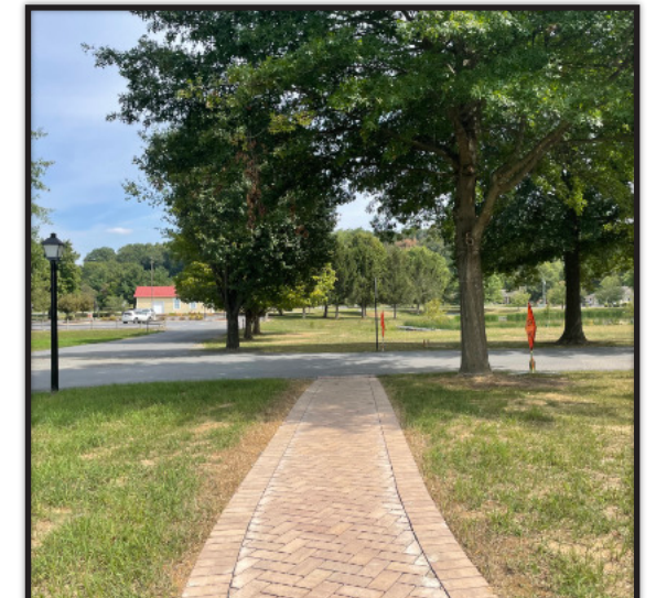
Construction of the Gen Oak Connector was completed last summer.
