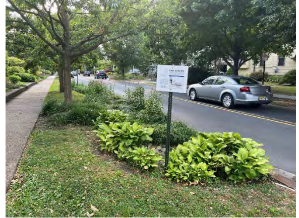
Figure 3: Rain garden in buffer between sidewalk and roadway designed to capture stormwater runoff.
