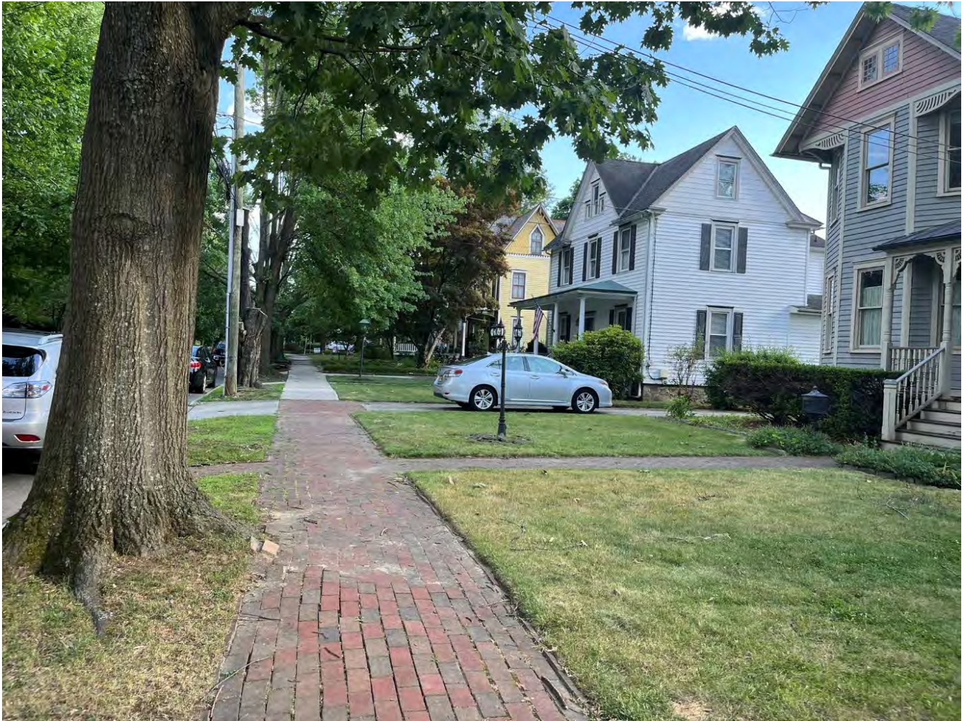
Figure 12: Roads within the Borough have nearly complete sidewalk coverage using a variety of materials. Some sidewalks are uneven due to deterioration or tree roots.
