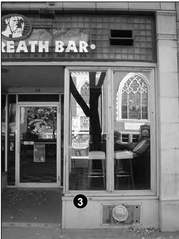
Fig. 5-83: 449 Main St. Bare lumber framing for the storefront windows is not in keeping with historic designs.
