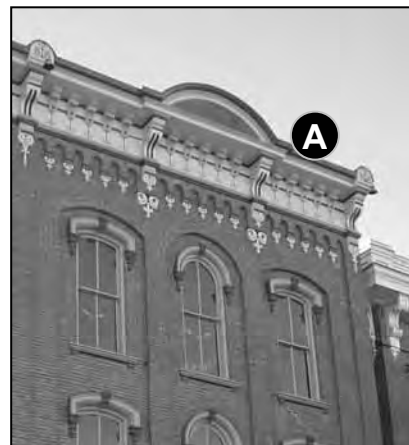
Fig. 5-74: 113 South St. The cornice of a multi-story building can be its most impressive design element, and is often where most color is used.
