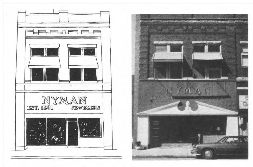
Fig. 5-85: On this storefront, the existing sign is too large, overpowering the building and its neighbors. The large colonial pediment detracts from the store name and is inconsistent with the building's architectural style. Removing this element and the paneling that extends to the second-story windows reveals more of the building fabric. A better proportioned sign that reuses the individual letters from the earlier sign can be placed in this space.
