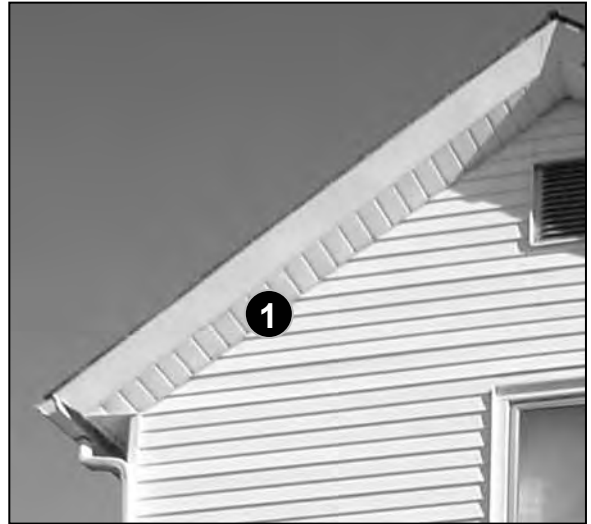
Fig. 5-33: 115 McKinley St. Vinyl siding hides the original wood trim that gives a façade definition and scale.
