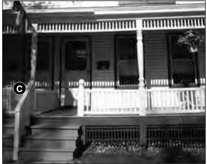
Fig. 5-4: 202 Main St. The front steps and railings up to this porch are similar to the style and character of the porch overall, and are painted to match. The underside of the porch is concealed with grillwork which allows the structure underneath to breathe.
