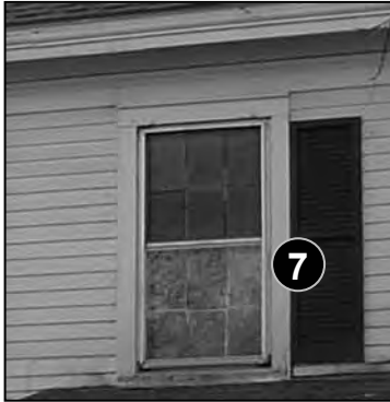
Fig. 5-22: 105 Holden St. Window shutters should be used realistically and consistently on a façade. The imitation window shutters like the one shown here are often seen used on only one side of a window, or on alternate sides of a pair of windows. Such installations are not historically accurate.
