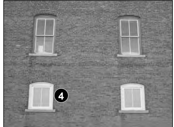
Fig. 5-26: 198 North St. The original arched top windows have been replaced with smaller, flat-top windows, and don't match from the second to the third floor.
