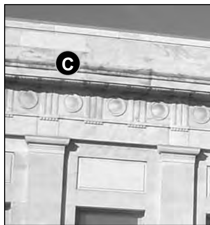
Fig. 5-32: 118 South St. Light colored stone surfaces such as this often need to be cleaned, but the cleaning process should never permanently change the appearance of the materials.
