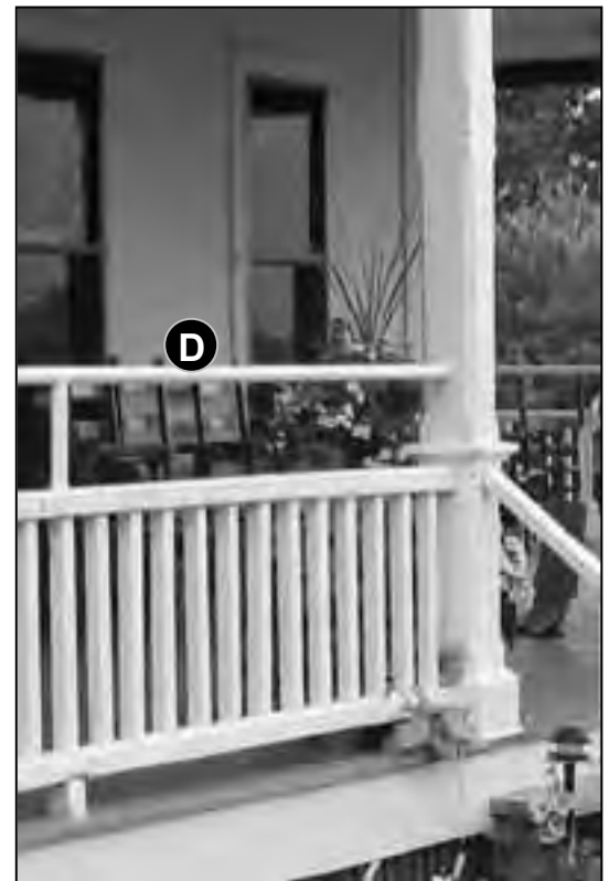
Fig. 5-2: Grand Isle Lake House, Grand Isle, VT. Original porch railings were very low, but new pipe has been added along the top to meet code requirements while still preserving the original scale of the railing design. Photo by Meg Cambell.
