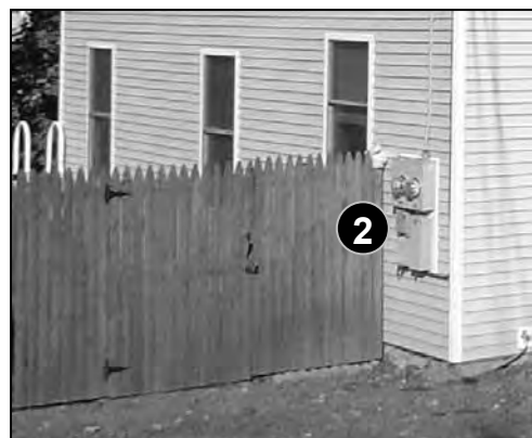
Fig. 5-63: Corner of Weeks & Jefferson. Although the electric meter has to be accessible, it doesn't need to be so visible.
