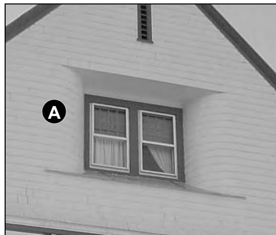
Fig. 5-30: 124 Elm St. Original curved shingles are used here to highlight the sculptural nature of the façade enclosure.
