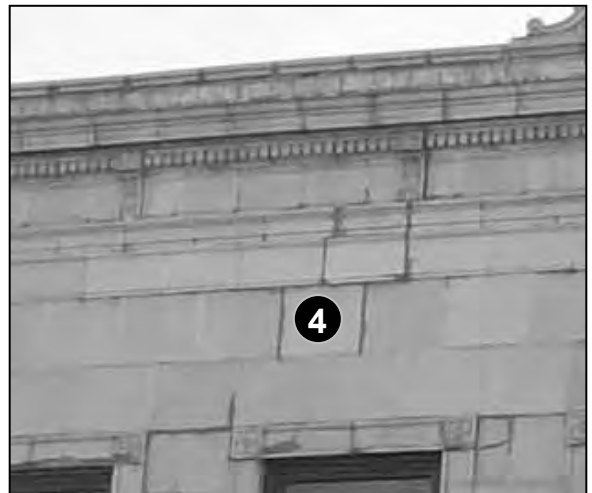
Fig. 5-35: 449 Main St. Joint repair which uses the wrong mix or mortar can result in highly visible joints. Be sure that test-mixes are tried before real work commences.
