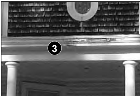
Fig. 5-53: 133 Elm St. The wood trim here is showing signs of moisture damage, and will get worse if left un-repaired.
