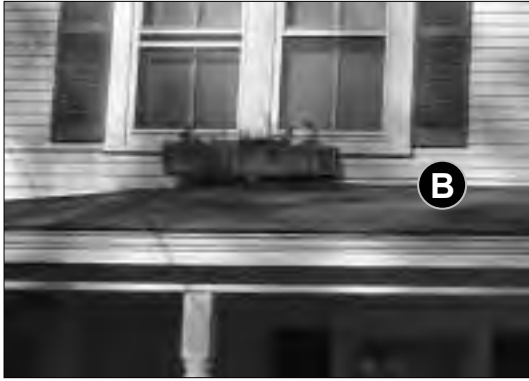
Fig. 5-3: 206 Main St. Porch roofs should be flashed properly and kept at least 10" below any windows to help prevent snow and water build-up at the window sill.
