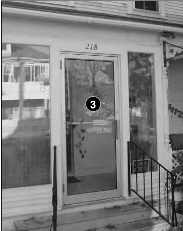
Fig. 5-12: 218 Park St. The commercial storefront door shown here is not appropriate on a residential structure.
