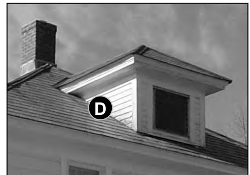
Fig. 5-44: 138 McKinley St. The shape of the dormer roof here matches the roof design of the rest of the building. If dormers or other changes to the roof are added at a later date, they should attempt to match the original design, and be placed out of view from the street.
