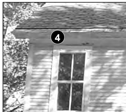
Fig. 5-55: 220 Silver St. The original copper eave flashing still remains along the edge of this roof.
