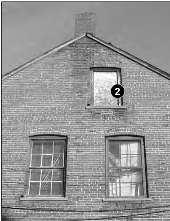
Fig. 5-28: 512 Main St. Windows that are no longer used should not be boarded up or filled in on the outside. Instead, the wall can be in-filled on the inside, leaving the existing window to remain on the outside.
