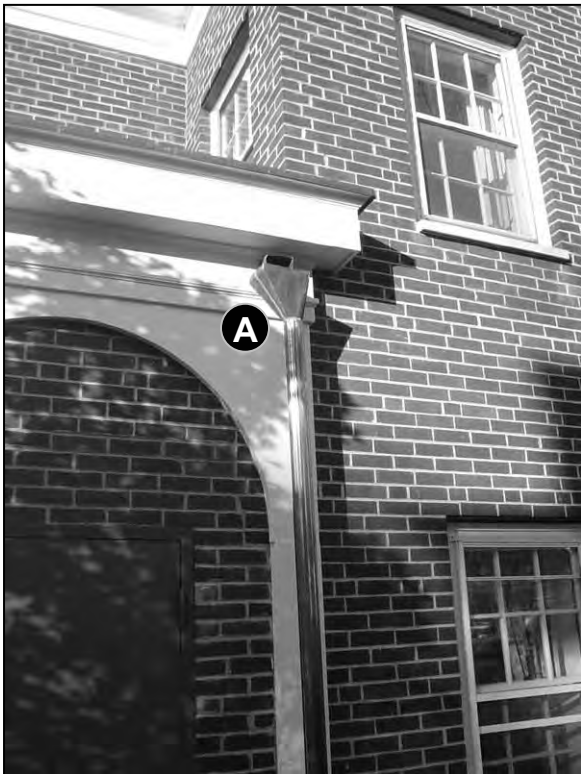
Fig. 5-54: 116 South St. A new copper downspout has been installed here to match the original materials.
