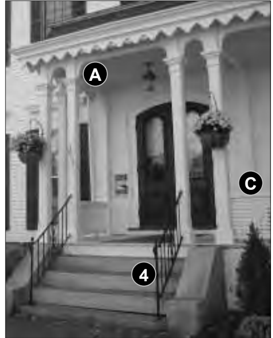
Fig. 5-1: 213 Main St. The ornamentation has been retained along the eaves, columns and porch railings, but the stair railings have been replaced with wrought iron.
