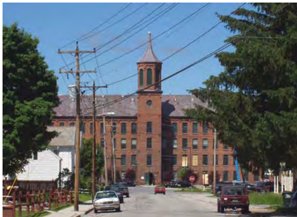
The Old Mill on Benmont Avenue is an important commercial building and connection to the town's industrial past. Its significance is emphasized by its prominent position at the end of County Street.
