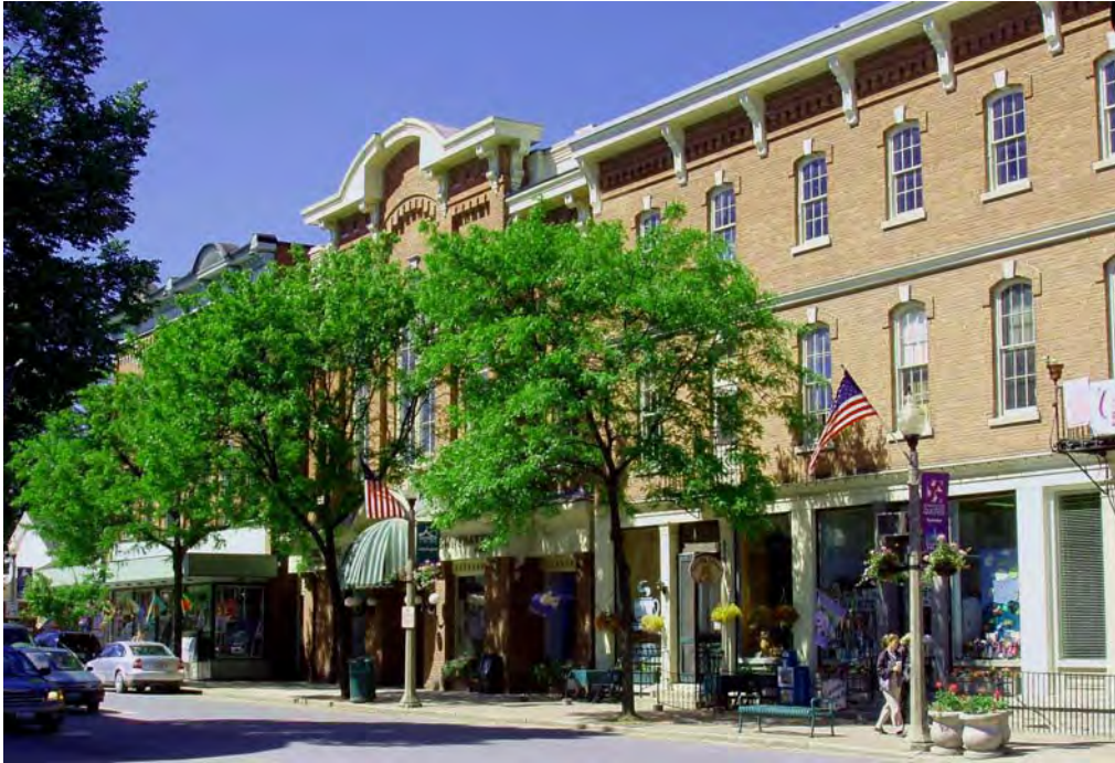
Downtown's historic buildings are enhanced by landscaping and appropriate site features such as attractive signs and period lampposts.
