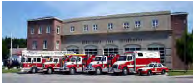
The Bennington Fire Department operates out of this impressive facility on River Street.
