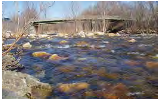
Restoration work along the Roaring Branch on the east side of town will improve water quality and floodplain management.
