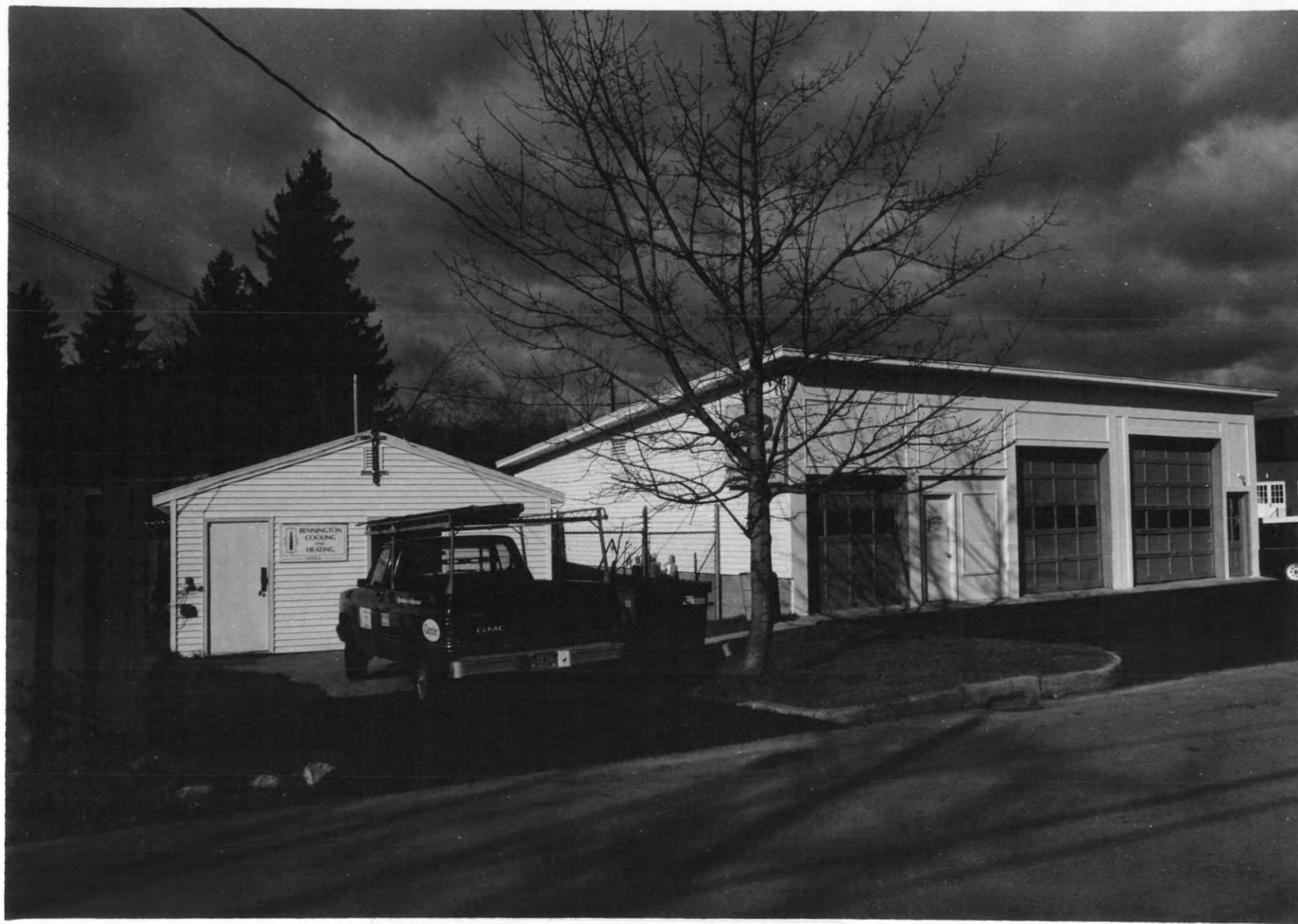
102 McKinley Street 88-A-281 Tracy Cuning VT Division for Hist. Preservation Bennington Co. Bennington 10/88
