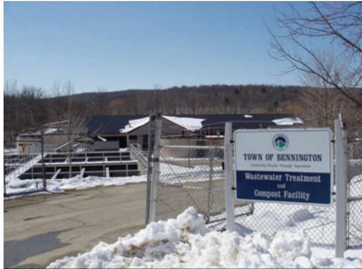
The wastewater treatment plant is the municipality's largest user of electrical energy.
