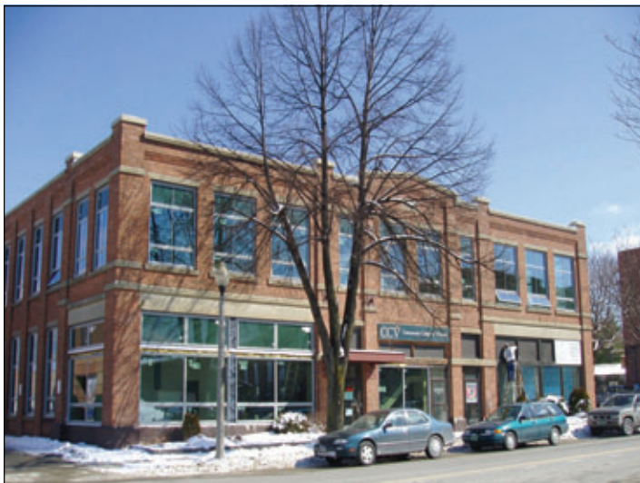
Numerous energy-efficiency measures were included in this office building, located on West Main Street, when it was renovated.
