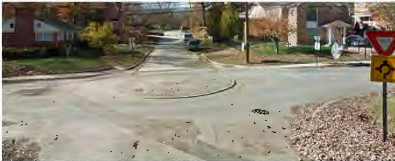
Traffic calming roundabout
