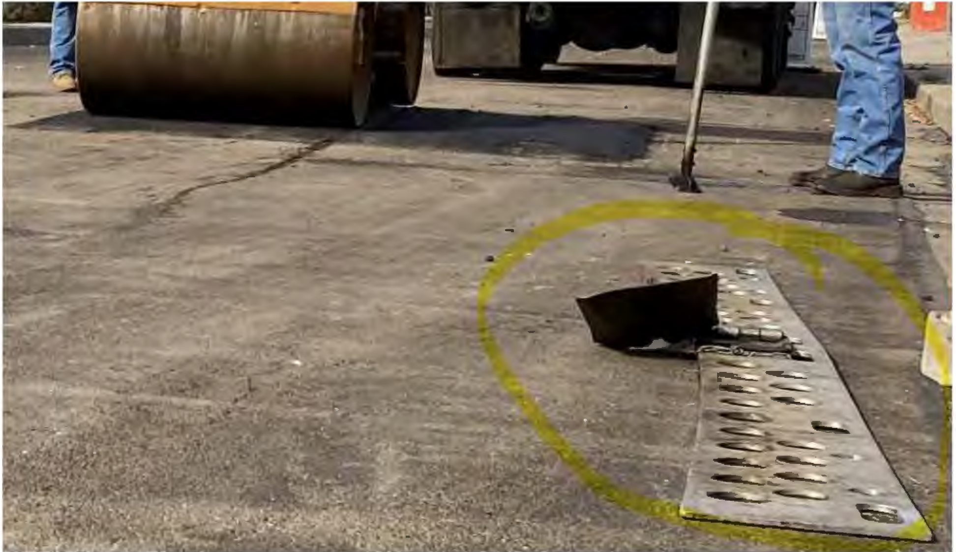
Figure 56. Speed Hump Construction Template.
