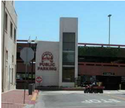
Glass-backed elevator shaft and cab
