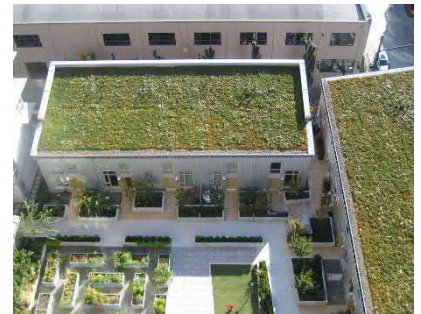
Green roofs help manage water run-off and reduce heat gain.
