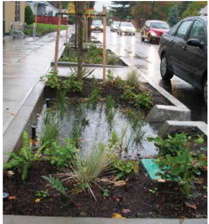
Stormwater infiltration planter between the street and sidewalk.
