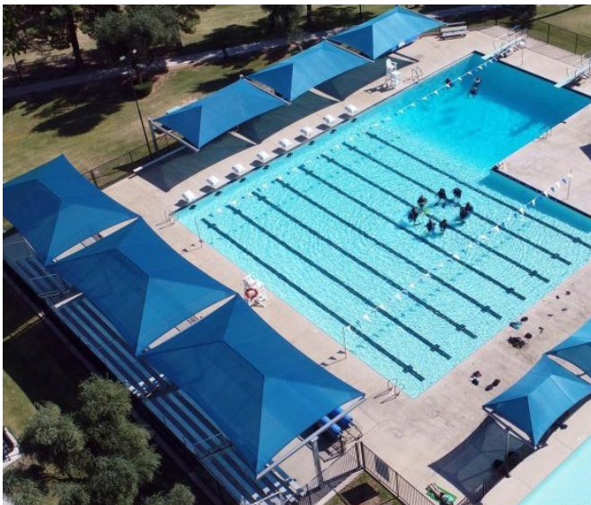
Bleachers example Source: shade-n-net.com/commercial/bleacher-shade-structures/
