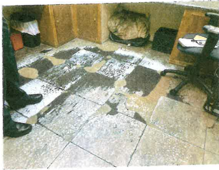
Front office floor
