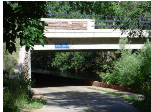
View from Tyden park of potential trail location under the M43 bridge (left). Boulder Creek trail underpass designed to accommodate occasional seasonal flooding (right, Boulder, CO).
