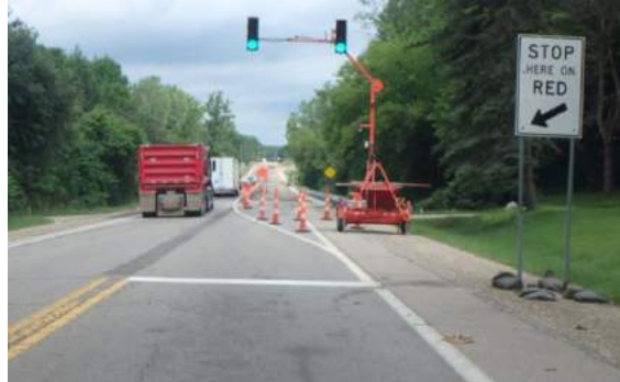
Reconstruction on M37 north of Crane Road.
