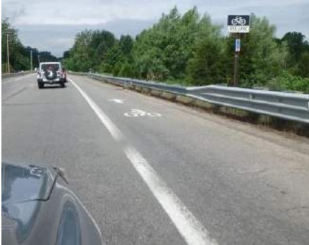
Crane Road bicycle lane.
