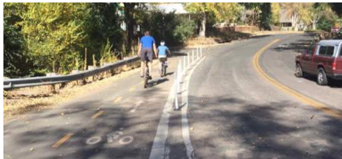
Example of a two-way shoulder side path, defined by paint and delineators.
