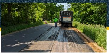
**ASPHALT - MILL & FILL** - Milling is an operation whereby the existing paved road surface is pulverized into small chunks, picked up and removed from the roadbed. After the existing asphalt is removed, varying depths of new hot mix asphalt is applied to create a renewed road surface. This tactic is most often employed when a roadway is nearing the end of its useful life cycle. Average life extension - 30-40 years
