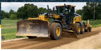
**GRAVEL - SPOT APPLICATION** - Spot application of gravel on gravel roadways involves the BCRC's crews evaluating the locations of habitual repair in order to prioritize locations to add gravel to the road surface. The process is completed when not enough funding is available to resurface the entire roadway and prioritization must take place.
