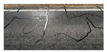
**CRACK SEAL** - Crack sealing is a process used on BCRC's paved road network countywide. Crack sealing involves blowing debris from cracks, covering the cracks with an elastic rubber over band, and spraying the rubber with a water mixture to quicken the set-up time. This process is used on roads with less cracks than roads that would normally be chip sealed, but both processes are completed in an effort to limit water infiltration into the road bed. Average road life extension - 2-3 years
