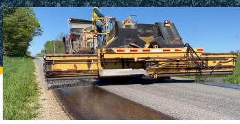
**EDGE & FULL SEAL** - Edge & full seal is a duplicated process where the outer 4' on each side of the road receives a chip seal. The edges are compacted and swept and then the entire roadway is chip sealed. This process adds additional protection to the outer sections of roadway, which are much more susceptible to damage. Average road life extension - 6-10 years.
