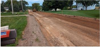
**FULL DEPTH RECONSTRUCTION** - Full depth reconstruction would be a smilar process to creating a new road or transitioning a gravel road surface to a paved road surface. Generally, the existing material is removed down to a depth between 11"-23". Sand is imported to create a sub-base, processed road gravel is placed to create a base, and hot mix asphalt is placed to create a new road surface. Average life extension - 30-40 years.
