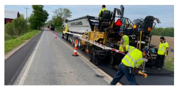
**ASPHALT - OVERLAY** - Overlaying an existing paved road involves placing an additional thickness of hot mix asphalt directly into an existing paved surface. This is a costly but very beneficial preventative maintenance measure if completed at the correct time in a road's life cycle. Average life extension - 20-25 years
