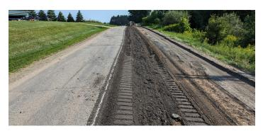
**ASPHALT CRUSH & SHAPE** - Crushing is an operation whereby the existing paved road surface is pulverized into small chunks, left in place and shaped in order to add structure to the road bed. In essence its creates additional gravel base beneath the new road surface. Once a road way has been crushed and then reshaped it is paved over with new hot mix asphalt. Average life extension - 30-40 years.
