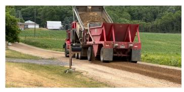
**GRAVEL - FULL-LENGTH APPLICATION** - The BCRC recommends a full 6" lift of processed 23A gravel on gravel road surfaces. When funding allows the BCRC crews will place a full road length lift of 6" of processed 23A road gravel. This process is certainly preferred by the BCRC, however, lack of funding often limits the ability to employ this process.
