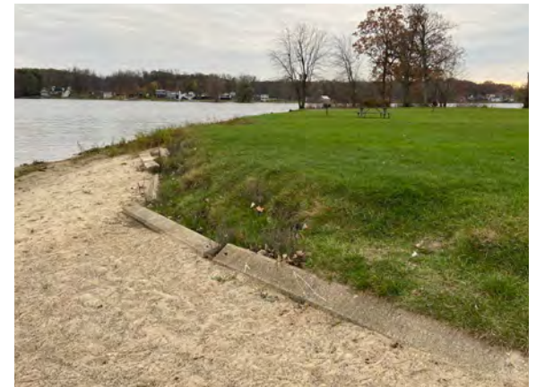
CONCRETE CURBING AT BEACH SAND AREA
