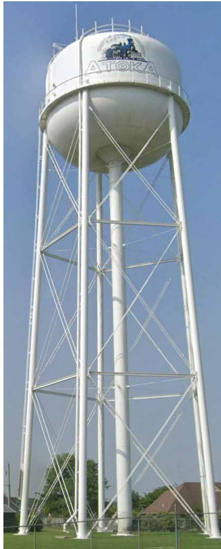
Atoka Water Tower
