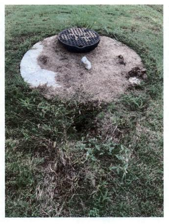
This is the current configuration of the above picture. It looks much better. However, the hole shown would indicate a hole in the manhole that water is entering in, and causing the loss of material that created this hole. The hole in the manhole needs to be repaired then the hole in the soil filled and seeded.
