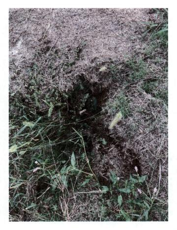
This photo shows erosion around the drain manhole shown above. All erosion should be repaired and permanently stabilized.
