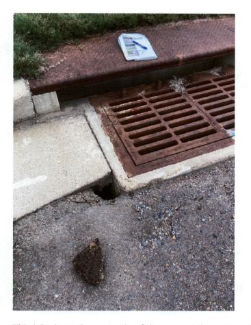
This inlet is on the east side of the cove at the east end of Sweetgum Lane. The hole in the picture is deep and extends under the curb and asphalt on the side and in front of the inlet. It appears that the water is getting into a hole other than the grate on top. This hole will need to be filled and the curb and asphalt repaired.
