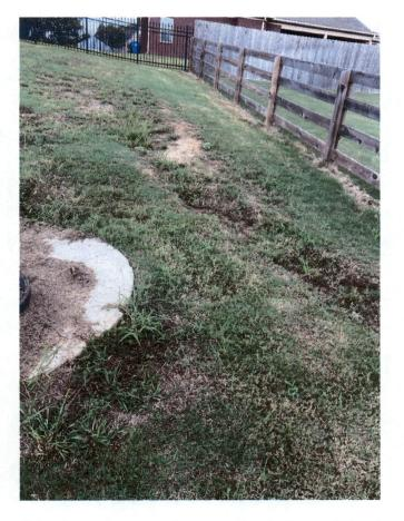
This photo shows erosion near the drain manhole above. All erosion should be repaired and permanently stabilized.
